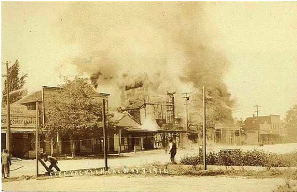
This fire in 1914 flattened all Front Street buildings between the granite Barudoni building, just out of the picture to the left, and Granite Drive, now Rocklin Road, to the far right. Today an insurance office and a church occupy two buildings to the far right. The rest of the area is still open space.
